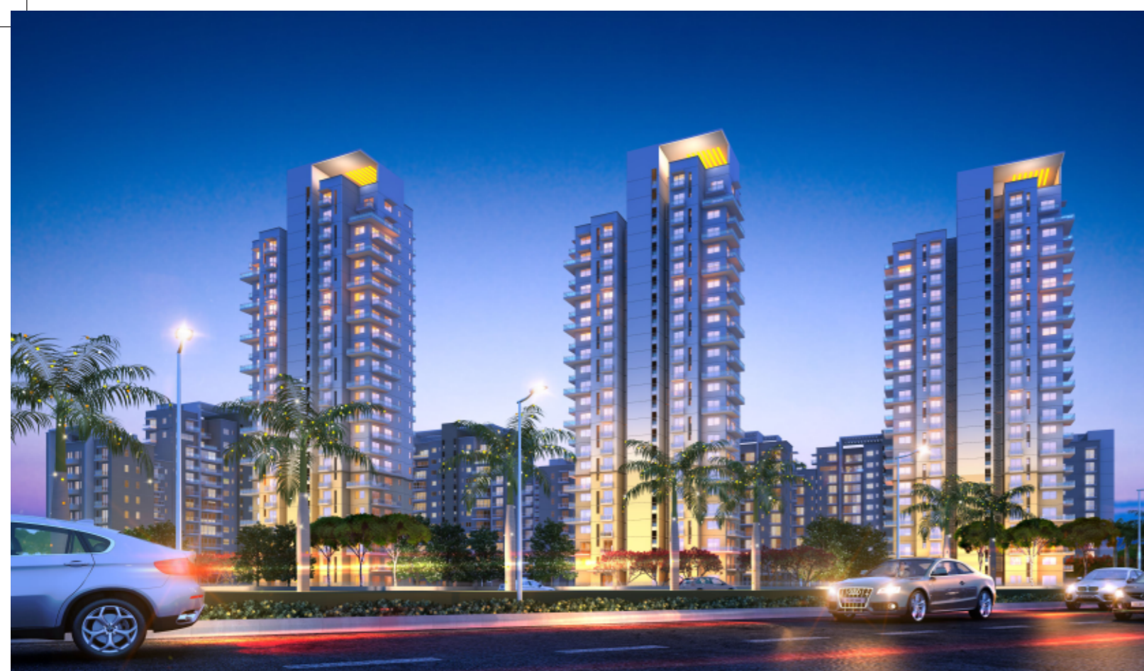
Located on National Highway NH 248BB
