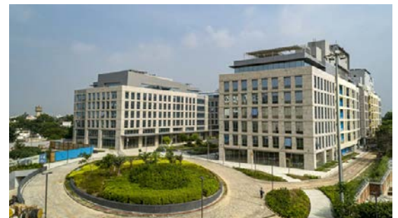
4 towers of One On One are ready for fit-outs
